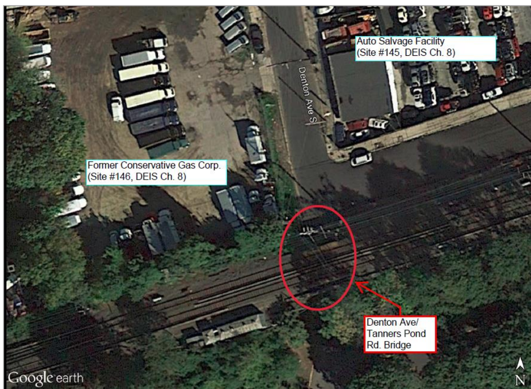
Figure 3.2 – Denton Avenue/Tanners Pond Road Bridge
