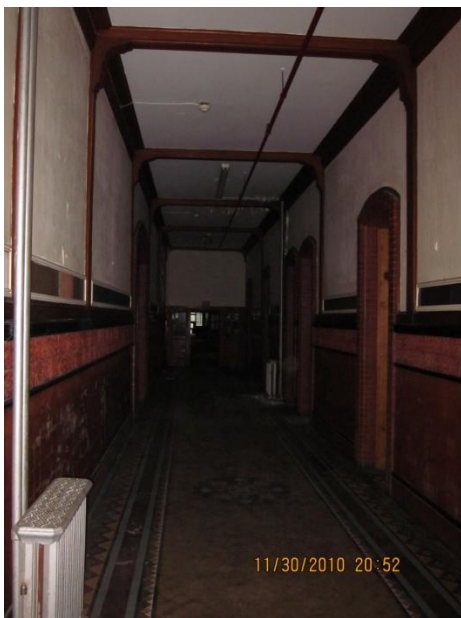
Typical Corridors. Corridor walls are structural and support the floor framing.
