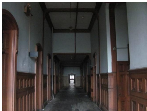
Typical Corridors. Corridor walls are structural and support the floor framing.
