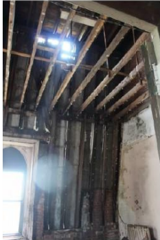
Figure 9: East Facade Roof Penetration - Interior Condition
