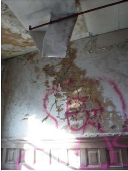
Deteriorated Room Finishes
