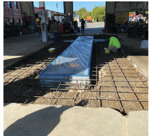
Replacing the Truck Lift in the Central Garage
