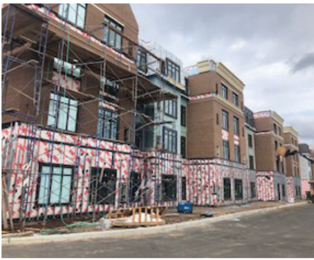
Ongoing project: Marriott Hotel at 700 Garden City Plaza
