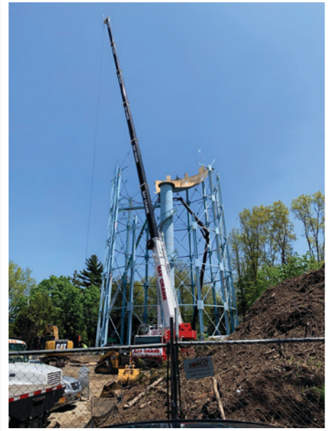
Dismantling of old water tower
