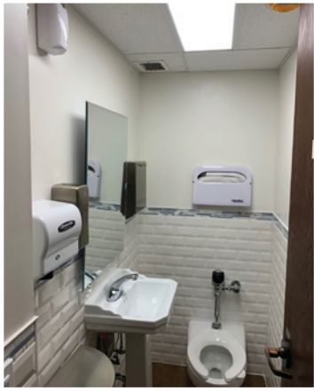
Garden City Library bathroom renovation
