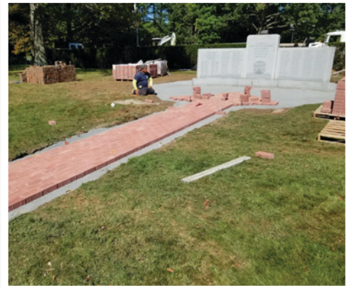
Garden City Firefighter monument restoration at Headquarters
