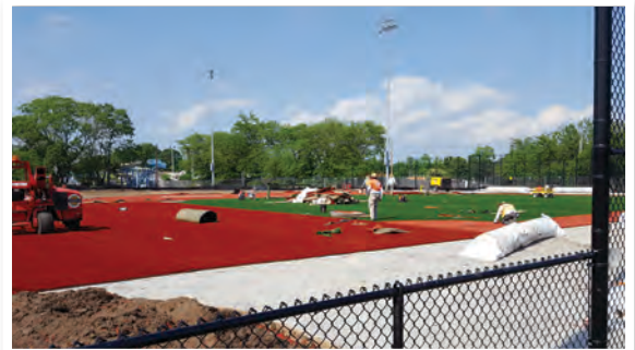
Construction commenced on fields 3 & 4 at Community Park, replacing infields with synthetic turf and outfields with new sod, installing new underdrain systems as well as new irrigation and fencing.
